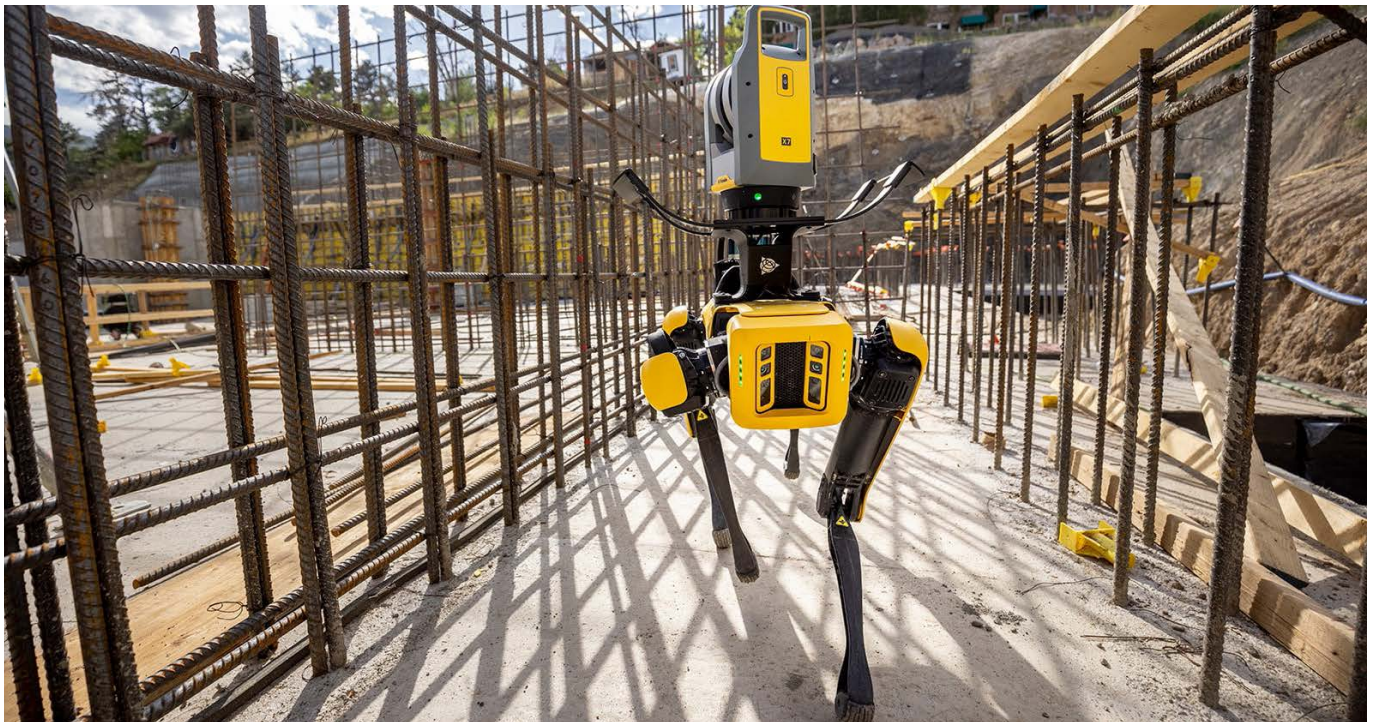
▲ 'Spot' the robot dog equipped with Trimble's X7 high-speed 3D laser scanning system. (Image courtesy: Boston Dynamics)
