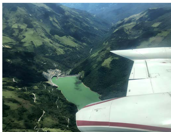
▲ Capturing data over the Ituango Hydroelectric Dam at 14,000ft (4,267m), in the mountainous terrain of Antioquia, Colombia.
