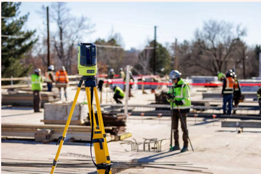
▲ Topcon's LN-1000i robotic total station set up on site to support construction layout and positioning tasks.
